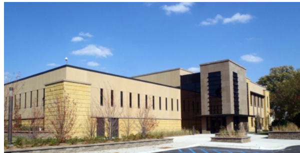
Houston County Justice Center exterior.
